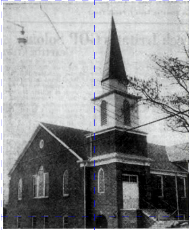
GROWTH CONTINUES — North Knoxville Baptist Church , Oldham Avenue at Worth Street, recently installed a copper steeple on its new $90,000 sanctuary which the congregation started using in November of 1953. Also, construction of an additional wing costing an estimated $25,000 was completed early this month.
